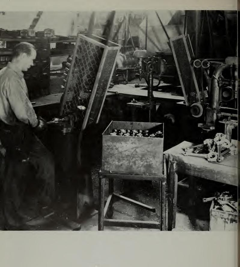
The cap is replaced on the rod using the original bolts and nuts, the removal of which was described in Picture 5. A power driven socket wrench is used in performing this operation.
